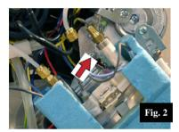
• Remove the mounting screw of the pipe heater.
