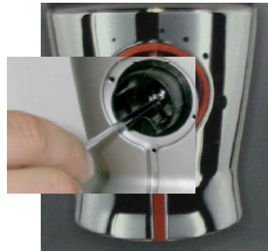
Remove the center screw and knob mount with a #1 Phillips head screwdriver.
