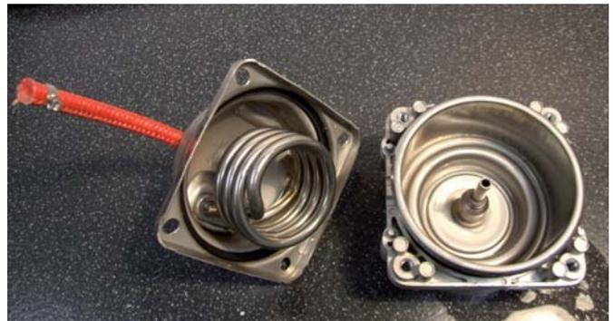
Check the internal condition of the boiler (limescale, any breakages, condition of the O-ring seal, etc.)
